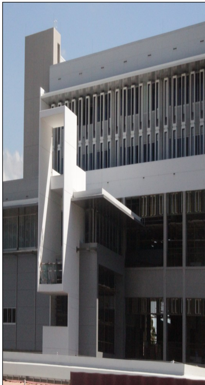
The new Court infrastructure at Waigani, Port Moresby.
